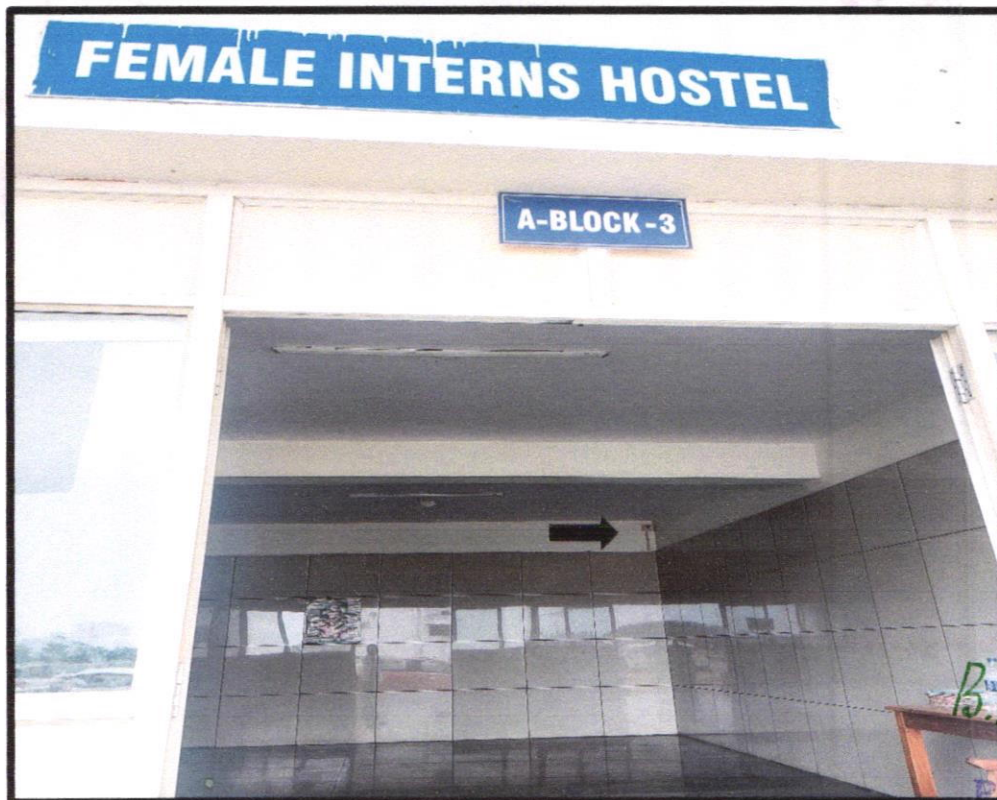
CCTV CAMERA IN FEMALE HOSTEL
